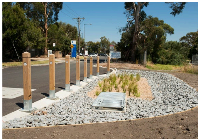
Example of blue-green infrastructure, Frankston (source: Melbourne Water, 2012).
