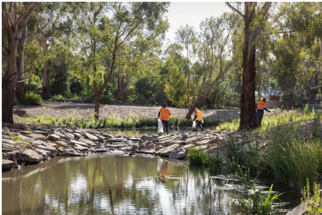
Example of channel modification, widening of Blind Creek (source: Melbourne Water, 2020).
