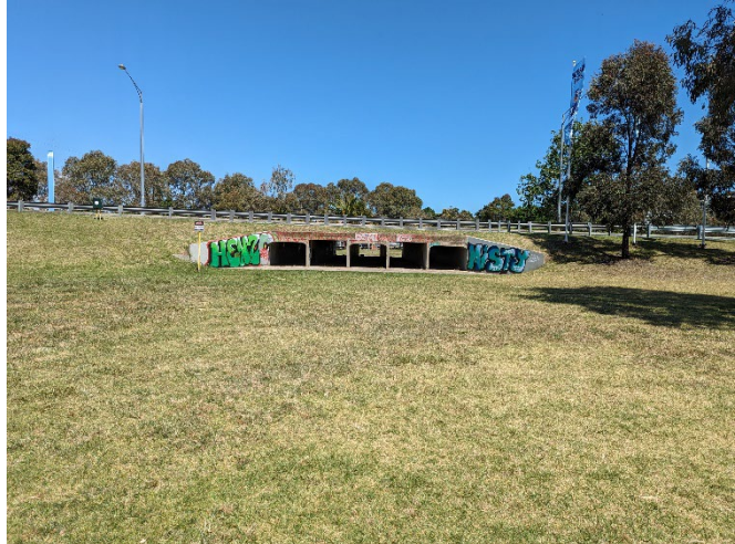
Example of flood relief culverts, Farnsworth Avenue, Footscray (source: Jacobs).
