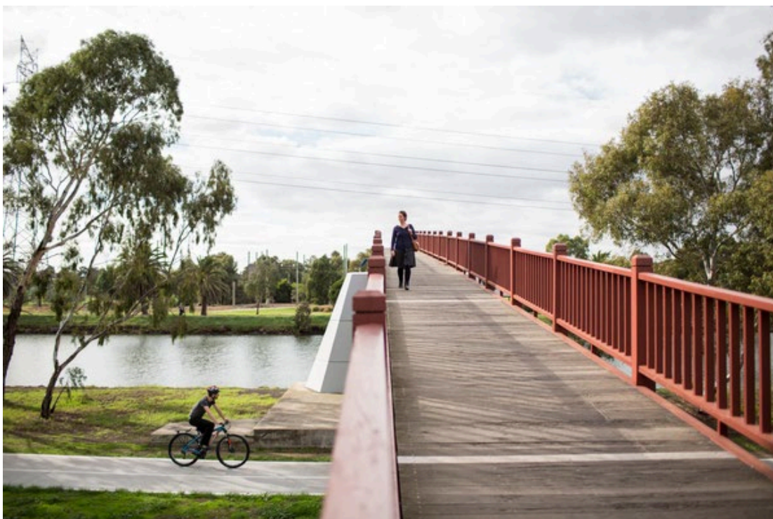
Example of a river bridge, the Maribyrnong River (source: Melbourne Water, 2016).
