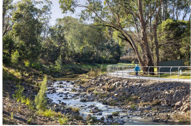
Example of a levee, Dandenong Creek (source: Melbourne Water, 2020).
