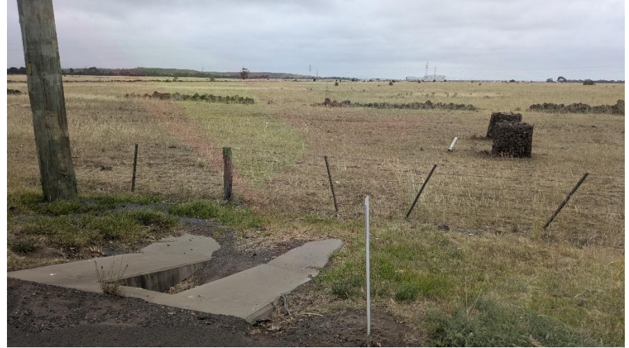
Figure: Culvert Crossing at Hopkins Rd between Boundary Rd and Middle Rd
