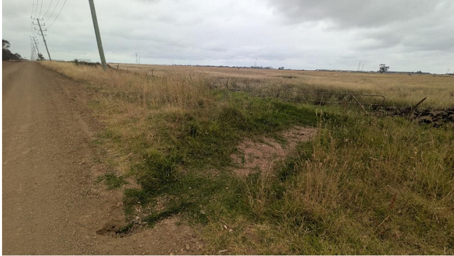
Figure: Skeleton Creek Culvert Crossing at Middle Road
