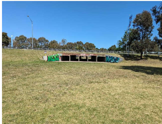
Example of flood relief culverts, Farnsworth Avenue, Footscray (source: Jacobs)
