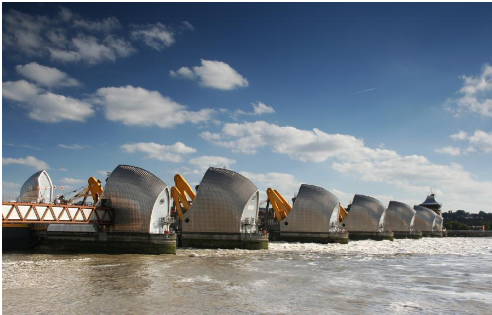
Example of an option that would fall in the 'Other' category, Thames Barrier, UK (source: Jacobs, 2025).
