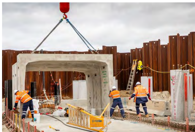
Concrete culverts and sheet piling
