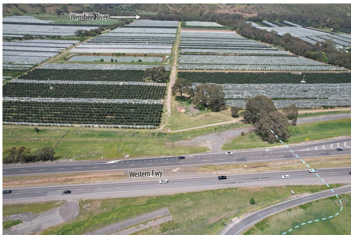
Figure 11. Looking south, a view of the Flanagans Run assessment area's main tributary crossing under the Western Freeway. The tributary's flow pathway to the Werribee River is currently unknown.
