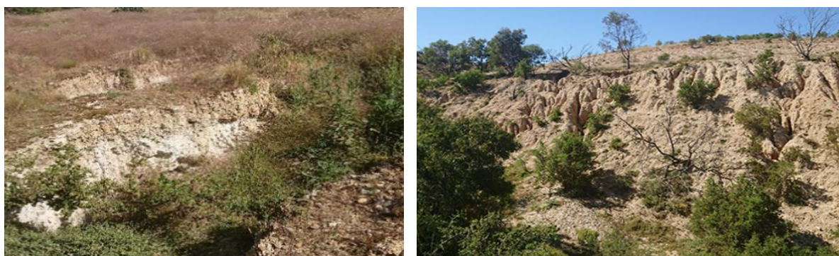
Figure 11 Tunnel erosion on the northern side of the drainage line at the base of the slope, immediately beside the waterway (left), looking downstream and across the waterway at the eroding cliffs on the southern side – beside the former quarry (right).
