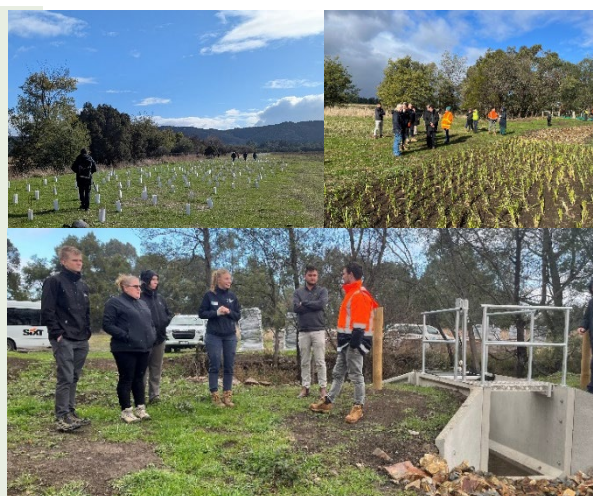
Images of the new flood gates and planting site at Yering Flats Photo credit: Rob Molloy and Elli MacDonald
