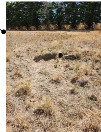
Waterway/ drainage channel with pipe.
