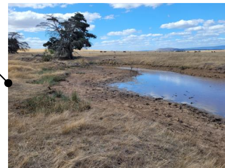
Photo looking NNE across dam
