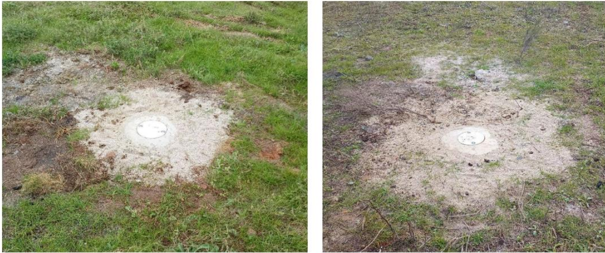
Figure 12. Left- GW01 final installation and, right- GW03 final installation.
